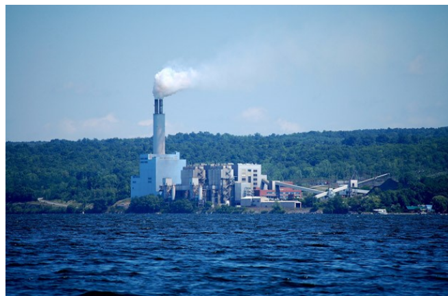
Cayuga power plant
